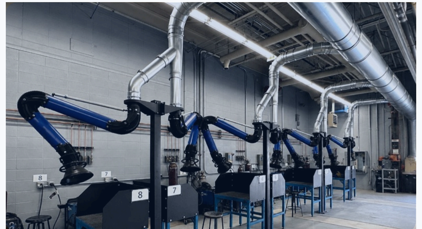
Modular extraction systems designed for expandable production environments.
